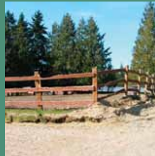
Before - Old, chewed on board fencing
