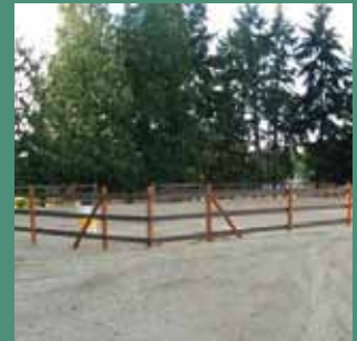
After - 5 1/2" Brown 3-wire Flex Fencing
